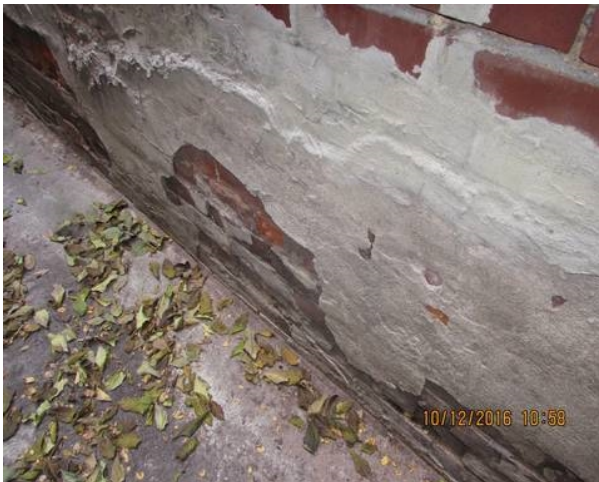
Deteriorated parging
