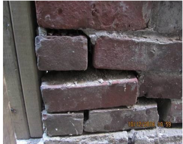
Mortar deterioration
