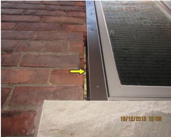
Opening at window
