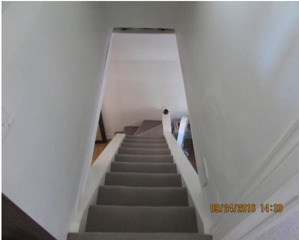
Missing handrail
