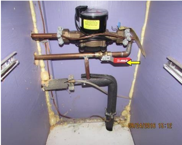
Water meter and main shut off
