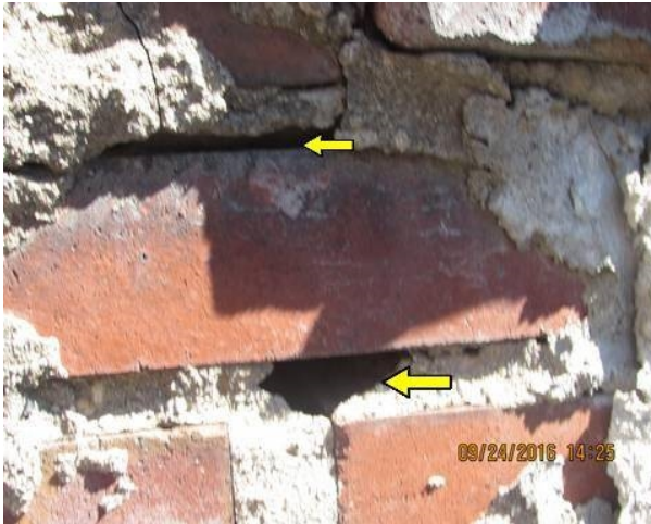
Deteriorated mortar
