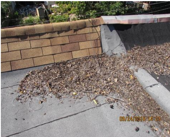
Debris on flat roof
