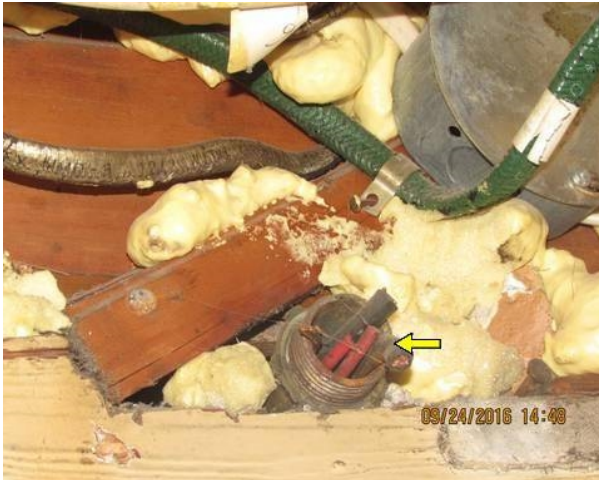
Exposed wires
