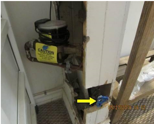
Water meter and main shut off
