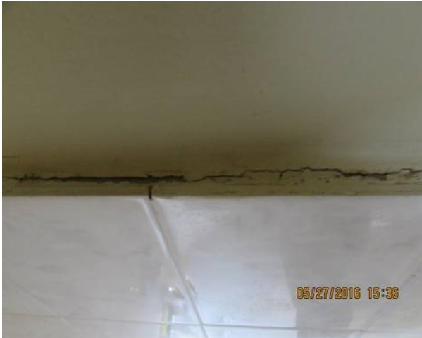
Deteriorating caulking
