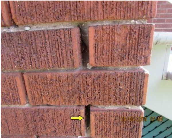
deteriorating mortar
