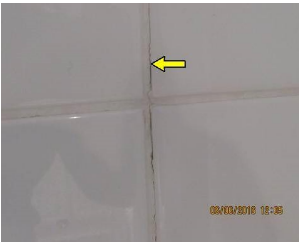
Cracked grout
