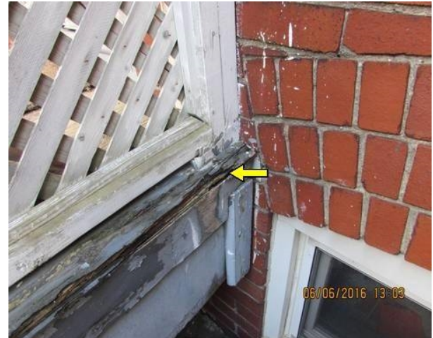
Deteriorating deck
