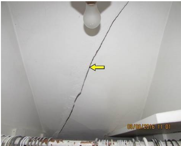
Cracked plaster
