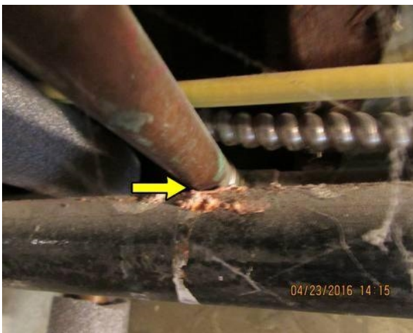
Dissimilar metals in contact
