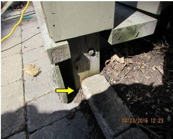
Wood to soil contact
