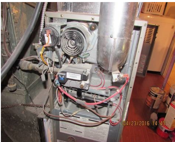
Mid efficiency furnace
