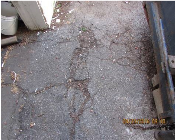
Deteriorating asphalt
