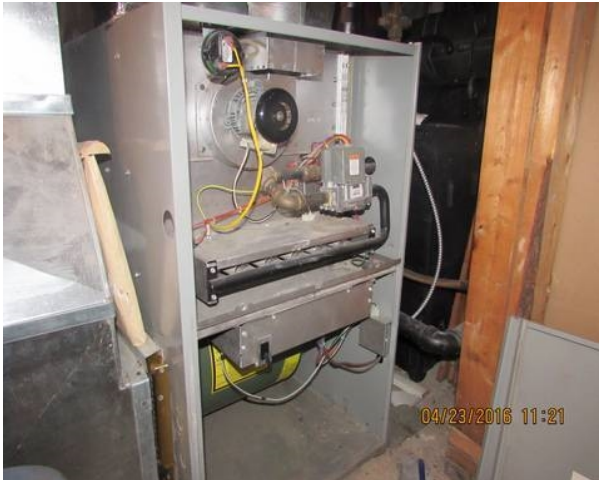
Mid efficiency furnace
