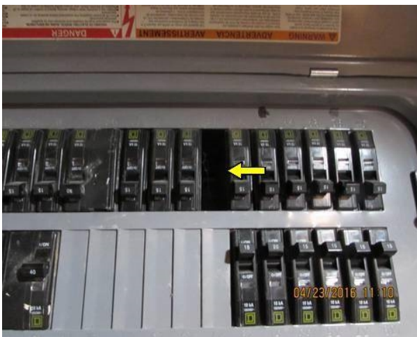
Openings to interior of panel
