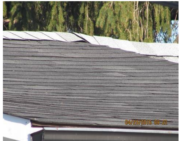
Shingles above east dormer
