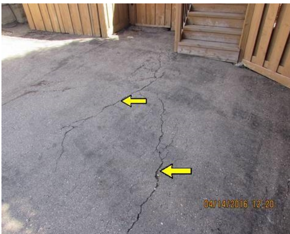
Driveway cracks
