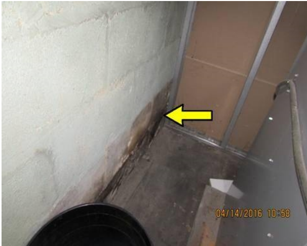
Staining on wall behind furnace
