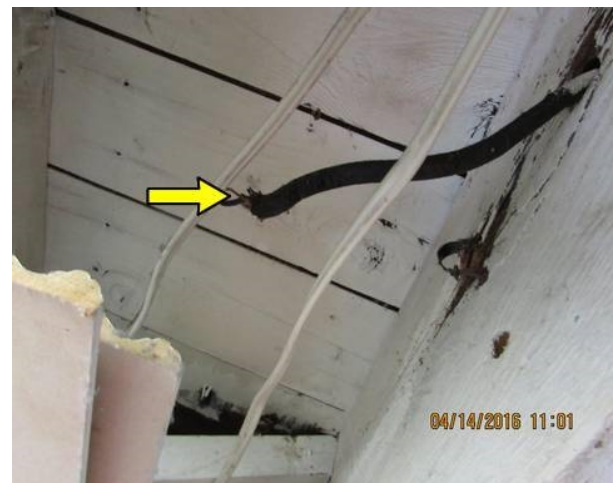
Unterminated and exposed electrical wire
