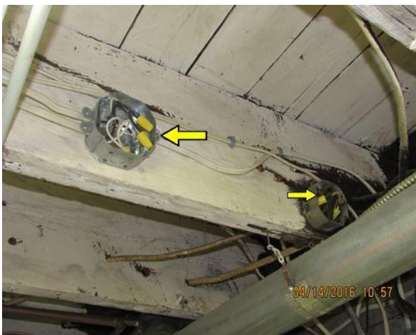
Missing covers on junction boxes
