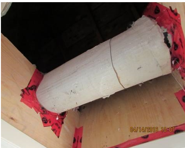
Possible asbestos material in duct insulation
