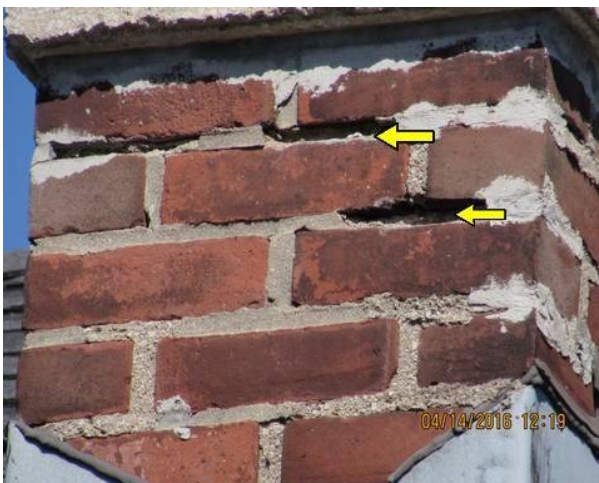
Mortar deterioration at abandoned south chimney
