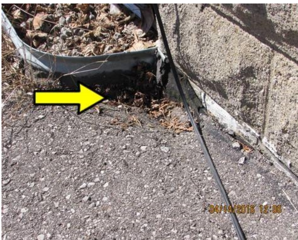
Grade slopes toward the foundation
