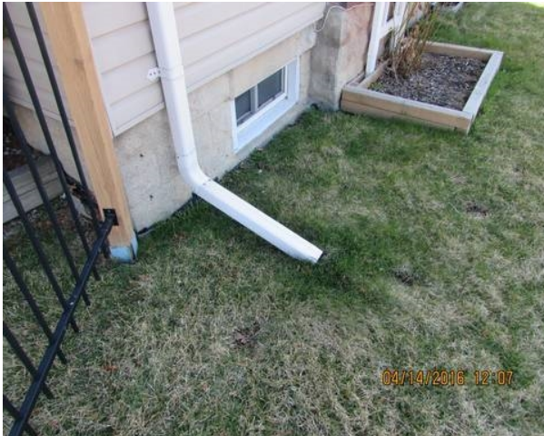
Downspout discharging to close to foundation
