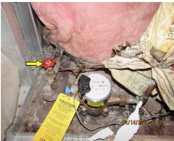
Water meter and main shut off
