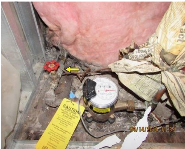
Missing ground clamp
