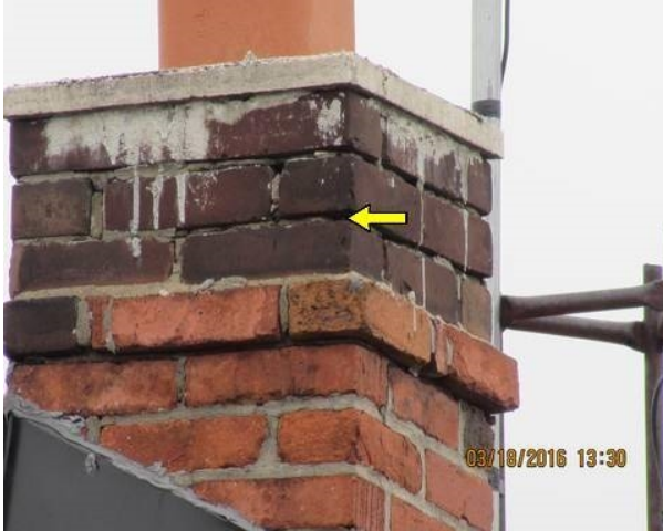
Mortar deterioration
