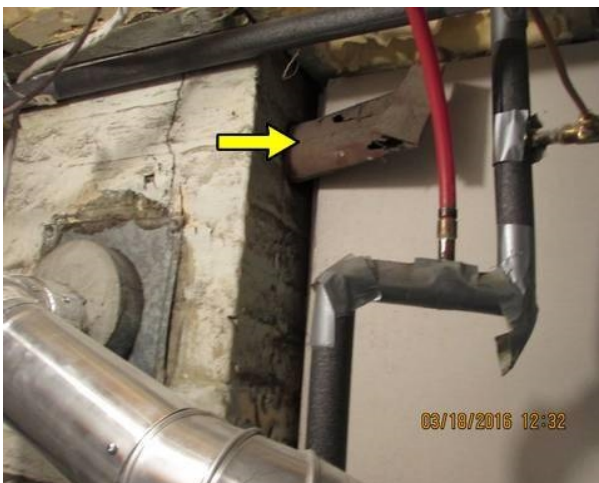
Remove old exhaust pipe and seal
