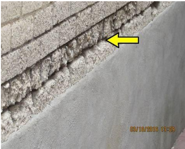
Brick deterioration
