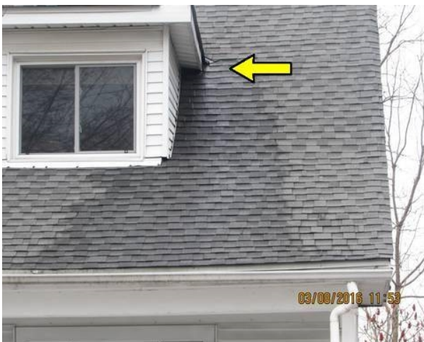
Large volume of water flowing off dormer
