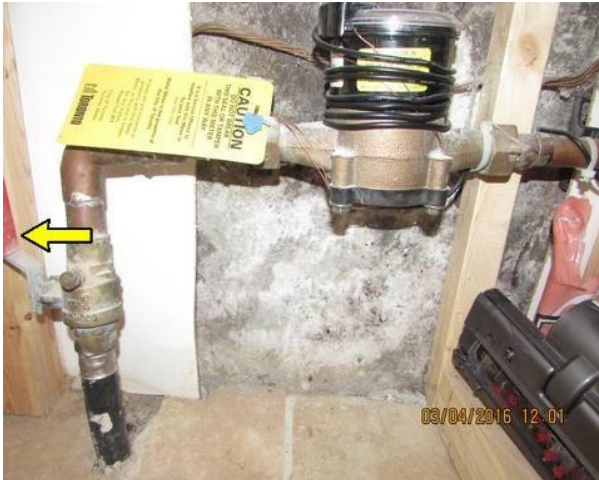
Water meter and main shut off
