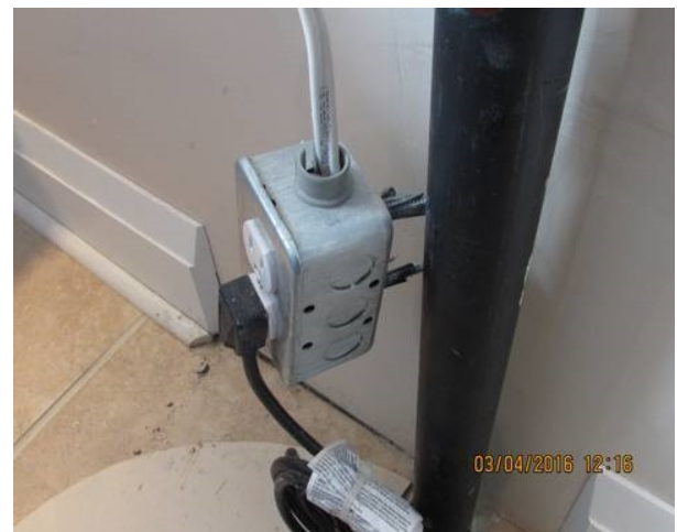
Unsecured electrical receptacle
