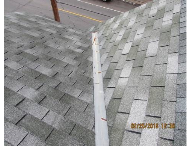
Shingles west side
