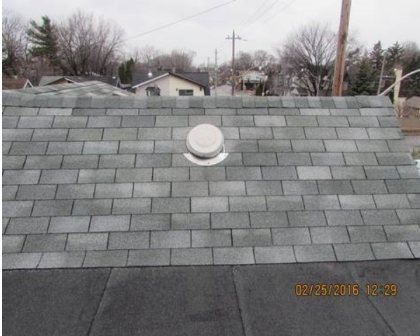
Shingles east side
