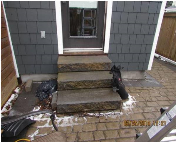
Missing handrail
