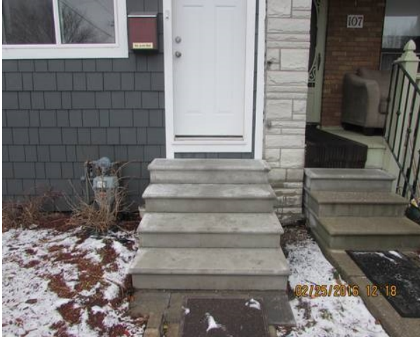
Missing handrail
