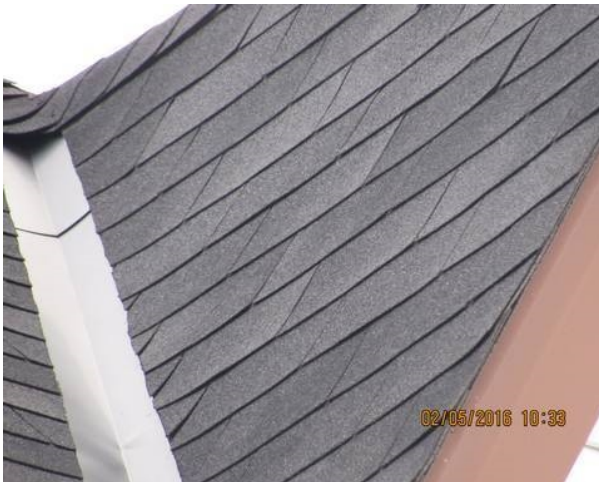
Roof covering west side
