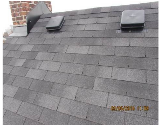
Roof covering on North view
