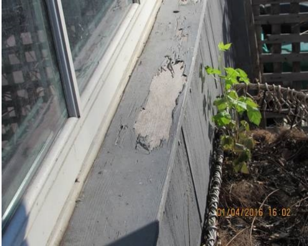
Paint wood trim
