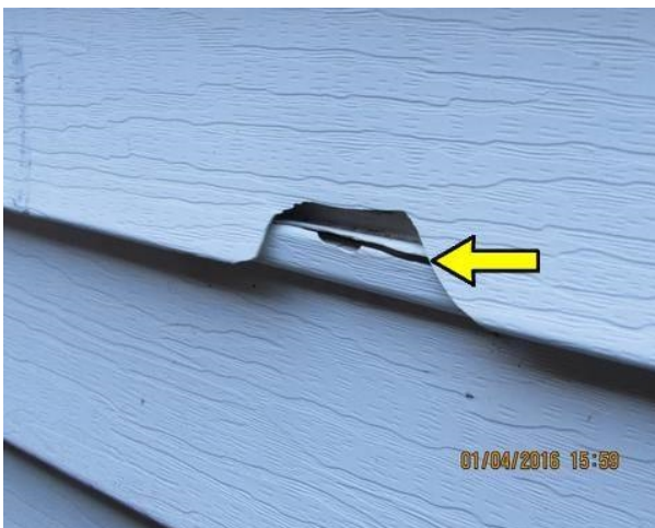
Damaged siding
