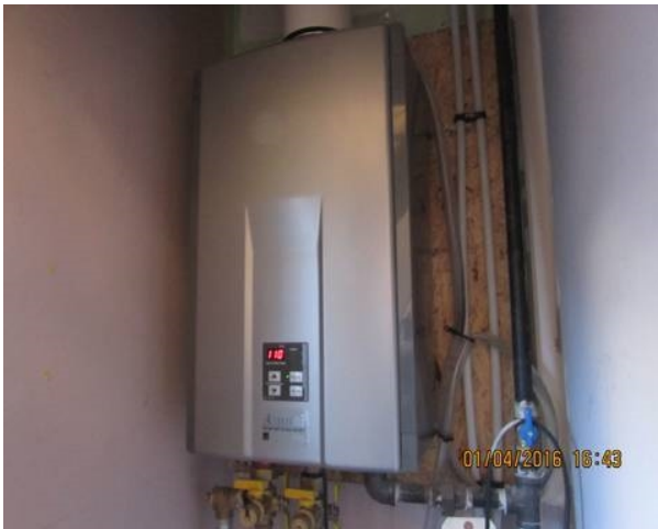
Tank less hot water system
