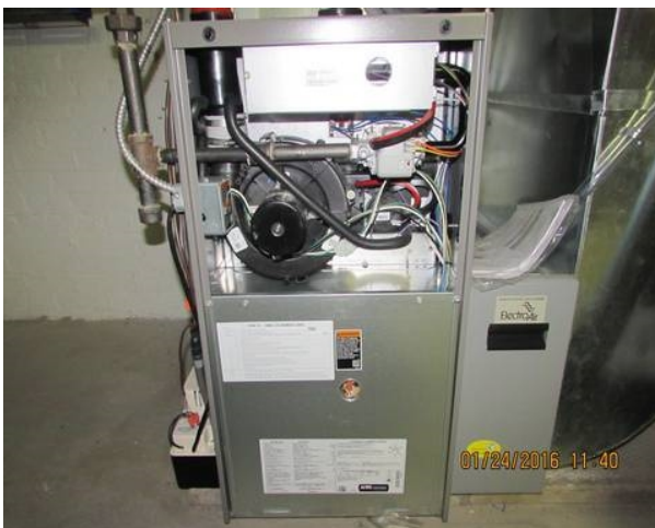
High efficiency furnace
