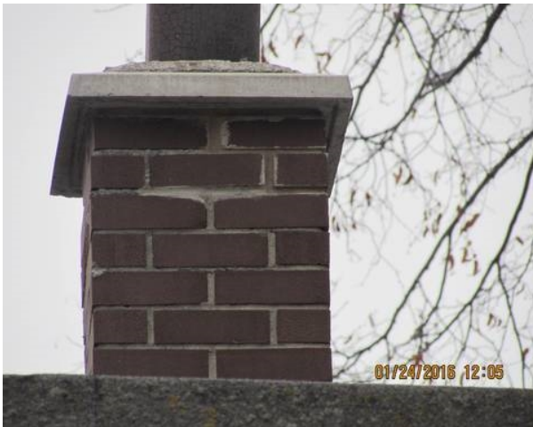
Abandoned chimney. Brick is in good condition.
