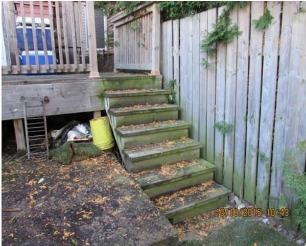
Missing handrail
