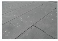
Bay(s): older slate though overall surface in good repair - monitor and repair as required
