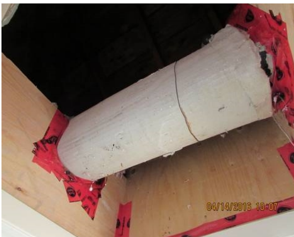
Unknown material used for duct insulation
