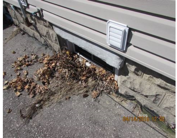
Basement window at grade
