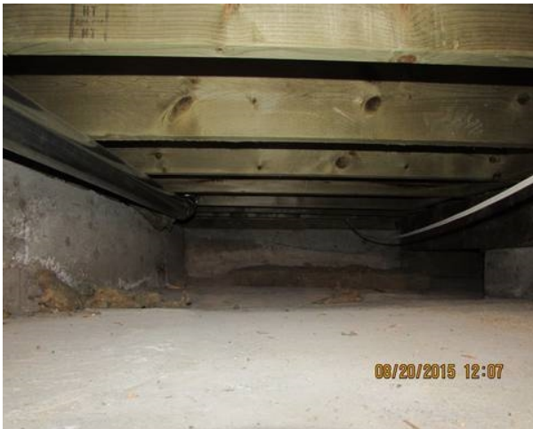
Crawlspace under kitchen
