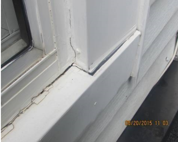
Caulk and seal around windows
