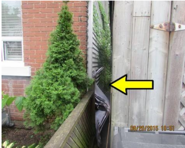
No access to west wall. Foundation not visible here.
