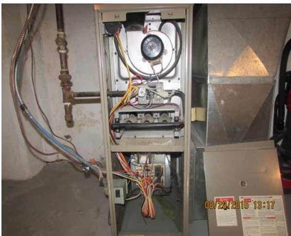
Mid efficiency furnace
